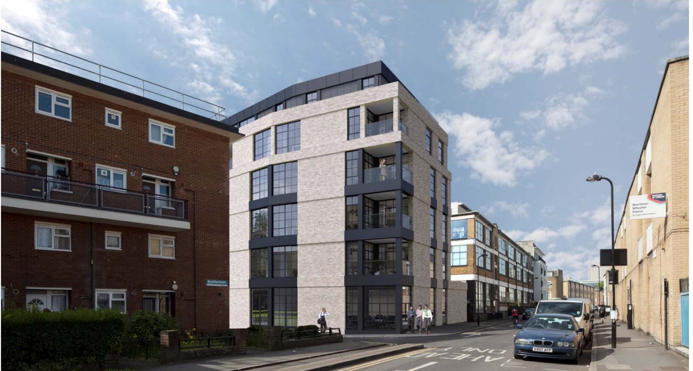
Eagle Wharf Road
